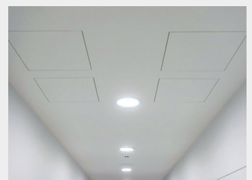
CEILING ACCESS PANELS
