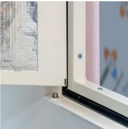
Hinge pin for easy positioning and door alignment
