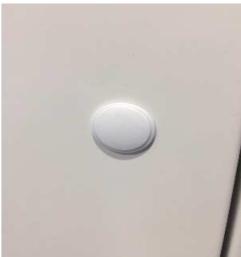
Metal Door Cap & Collar installed
