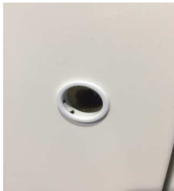
Metal Door Cap removed, Collar exposed
