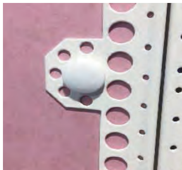
Plaster Board Bung installed
