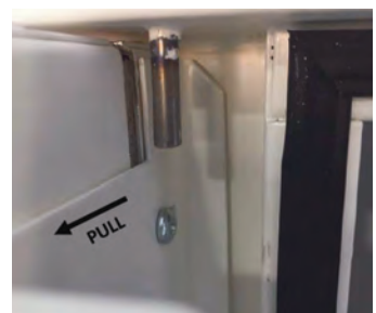
Remove pivot from panel and pull panel out of frame
