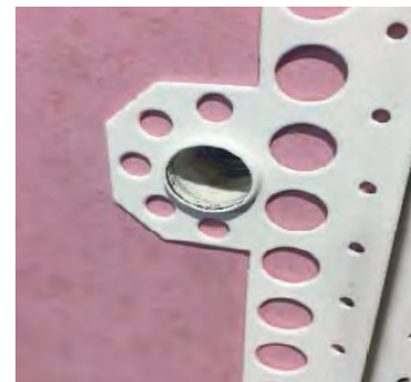
Plaster Board Bung Removed
