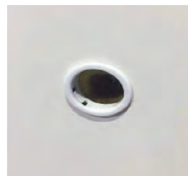
Metal Door Cap removed, Collar exposed
