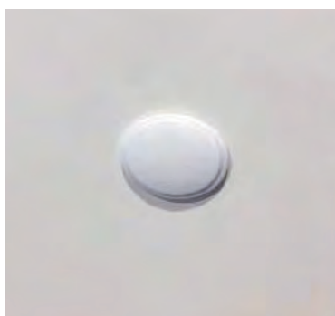
Metal Door Cap & Collar installed
