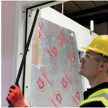
Position the spacer along the hinged side of the frame and door assembly.
