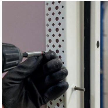
Face fix the beaded frame to the wall using suitable substrate screws. Ensure the fixings do not protrude past the face of the bead.
