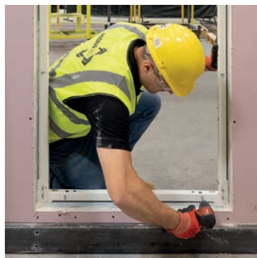
Secure the frame on all sides through all fixing points of the frame.
