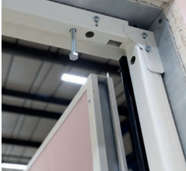
Insert the jacking screws top and bottom if they are not already fitted into the frame.
