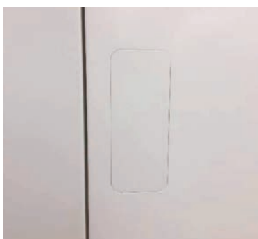
Cover installed flush
