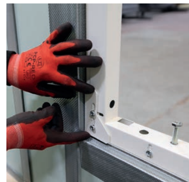
Lock the real bolts on the back of the frame ensuring the plates are pushed tight against the sub frame.
