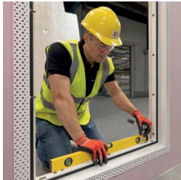
Adjust the position of the frame using the jacking screws to ensure it is aligned vertically and horizontally within the structural opening.
