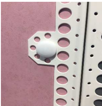
Plaster Board Bung installed
