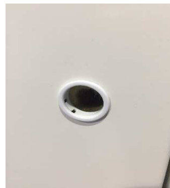
Metal Door Cap removed, Collar exposed
