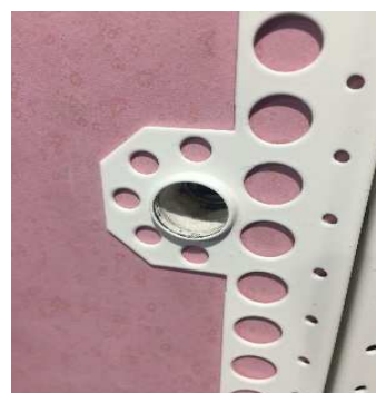
Plaster Board Bung Removed
