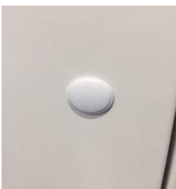
Metal Door Cap & Collar installed
